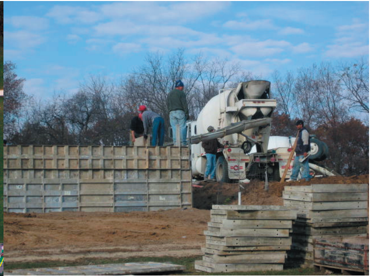
Digging the foundation and pouring the basement walls for Tall Oaks Lodge at Camp Quaker Heights
